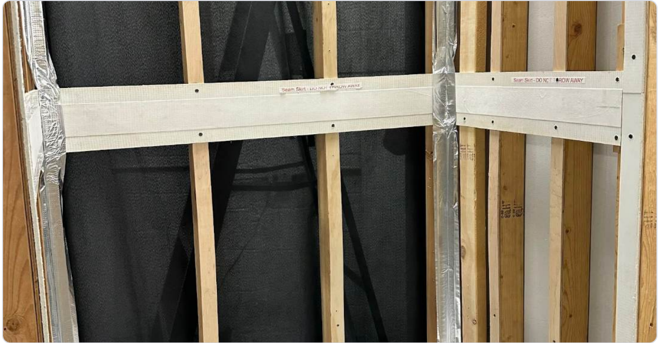
SKIRTING AND CORNER FLASHING IN PLACE, PAN FLASHING LAPPED FIRST.
