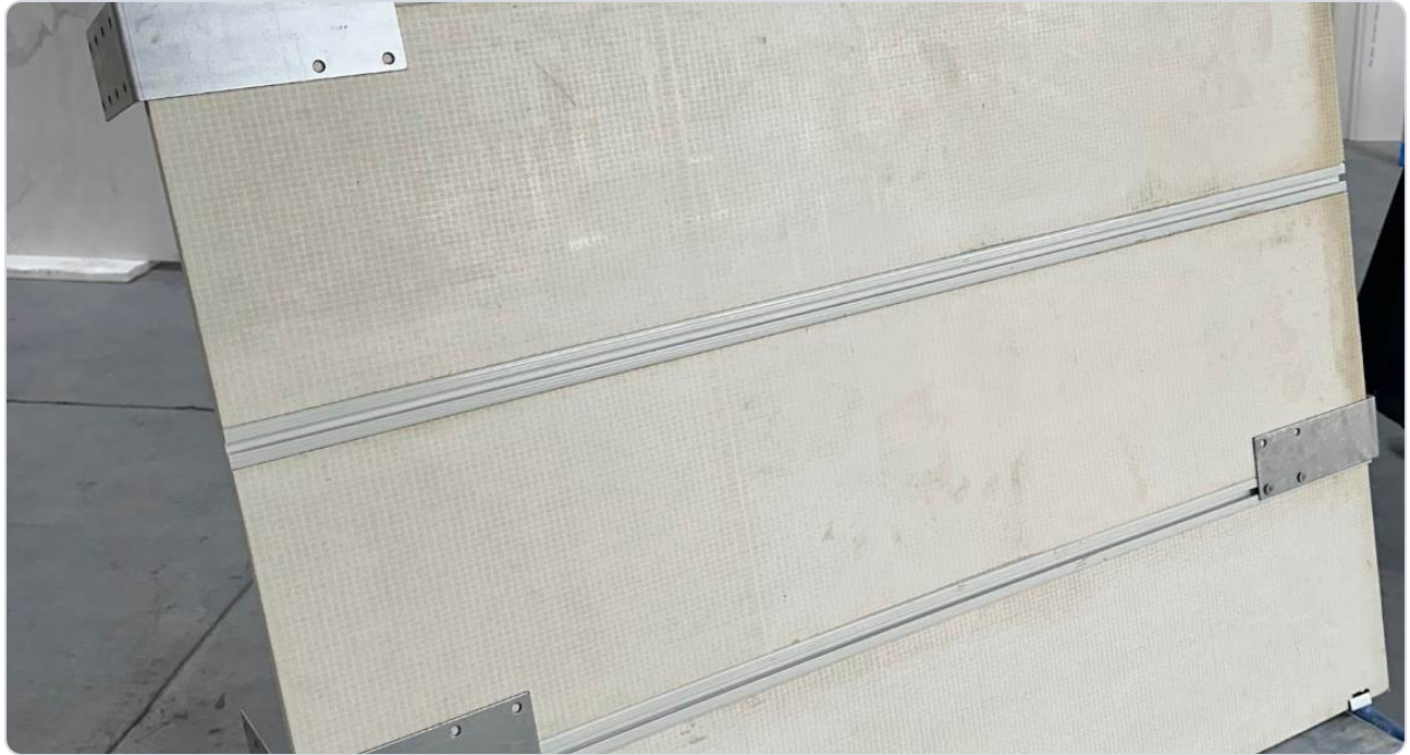
BACK WALL L-BRACKETS SQUARED AND SPREAD ON THE PANEL TRACKS.
